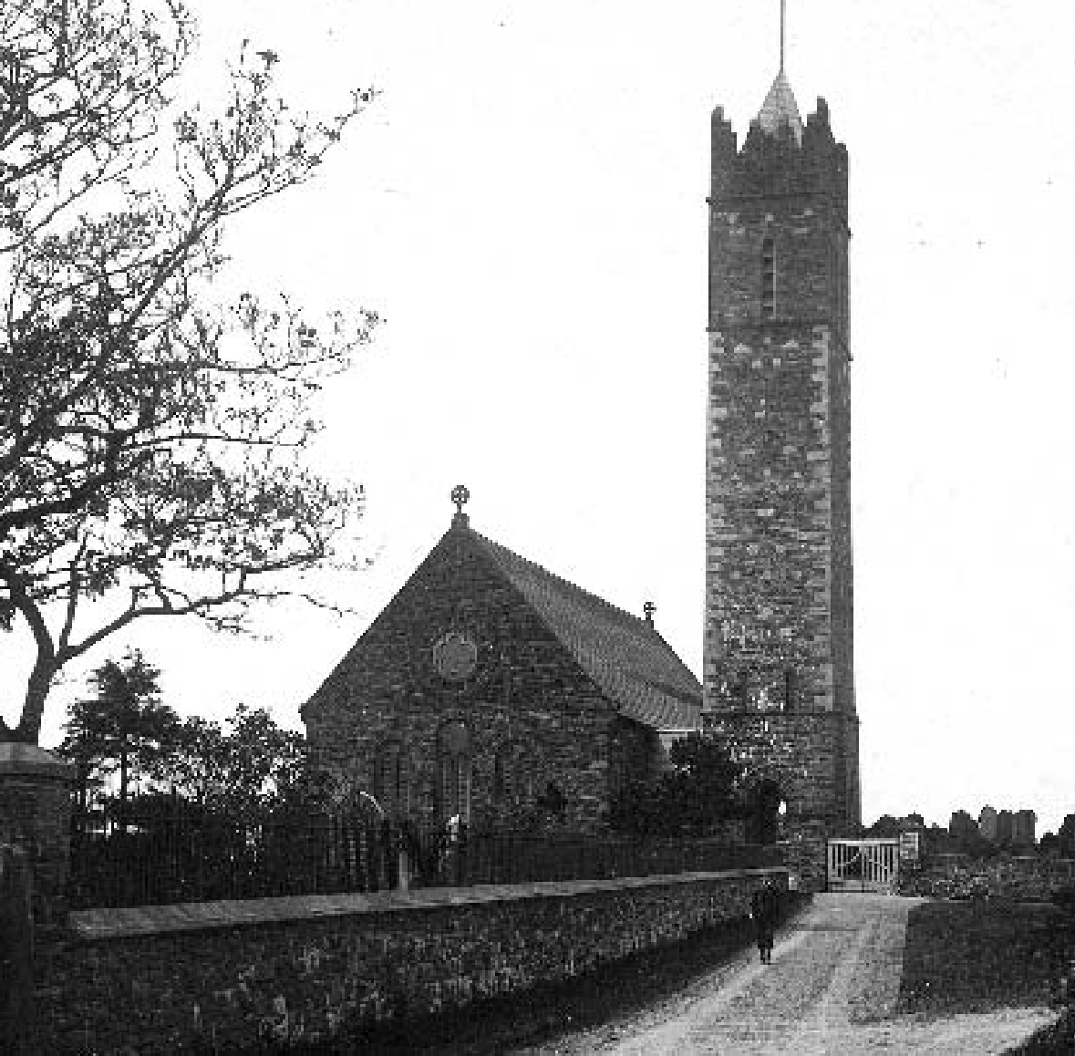
The RAF at Andreas During the Second World War the RAF's two airfields at Jurby and Andreas dominated the service and social life of Ramsey and the north of the Island. As this photograph shows, the fine tower on Andreas Church presented a hazard to low-flying aircraft before it was reduced to about half its height. (MNHL)
