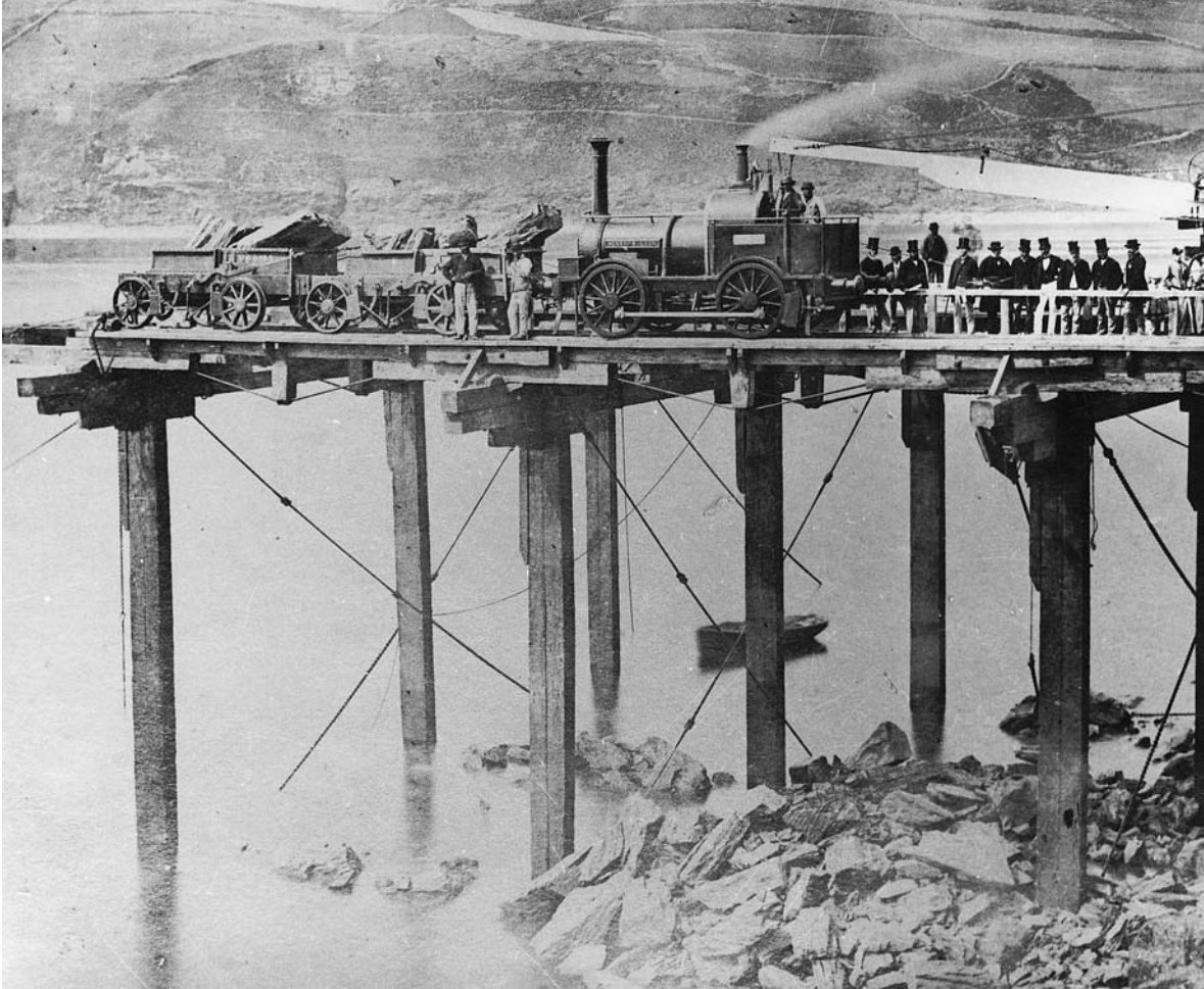
Port Erin Breakwater under construction. The building and financing of the breakwater was the subject of prolonged negotiations between the UK and the Manx authorities between 1861 and 1879. While other harbour projects undertaken during Loch's governorship proved of immense value to the Manx economy, the Port Erin Breakwater was subject to repeated storm damage and was finally destroyed in 1884.
